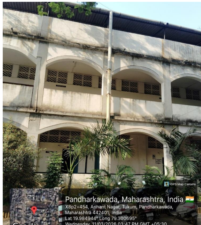
Figure 10- Rainwater harvesting structure in the college campus.
